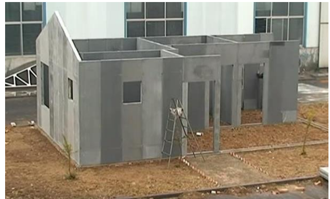
Fig. Load bearing wall with pre cast panel
