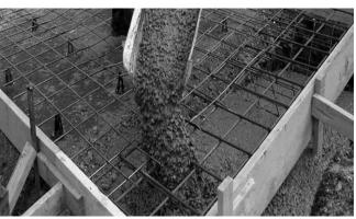
Fig. Geopolymer Concrete in Reinforcement
